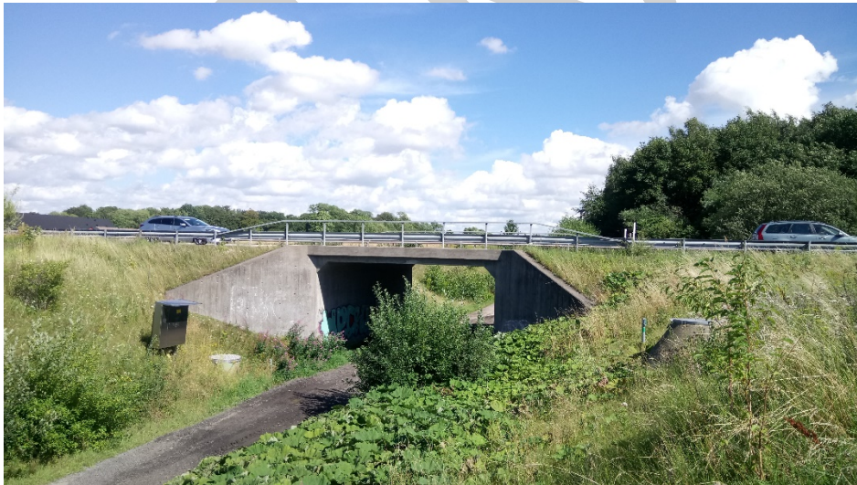
Figure 1. Bridge seen from the west. Photo taken in July 2017.
