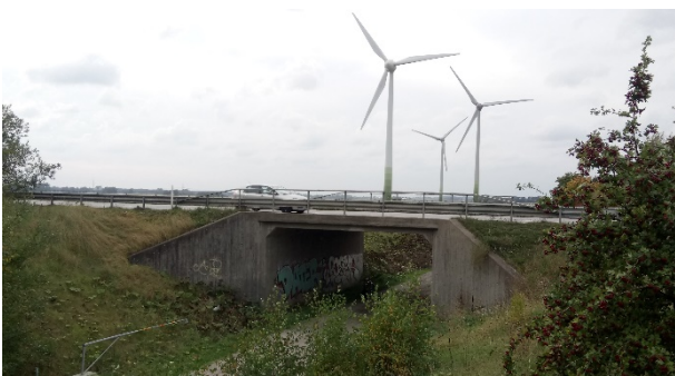
Figure 1. Bridge seen from the east. Photo taken in September 2017.
